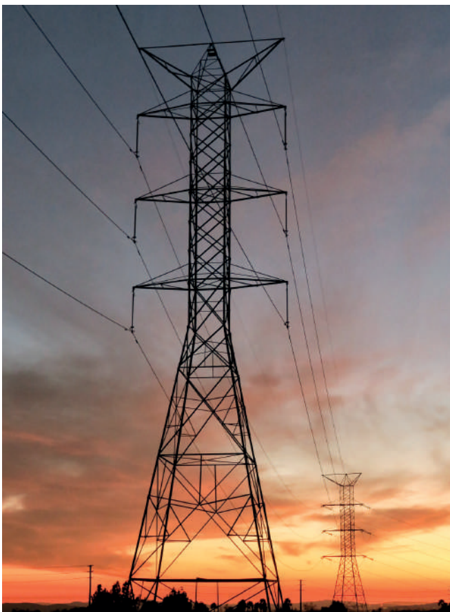
Image: Electrical energy is transmitted through high voltage electrical lines.
